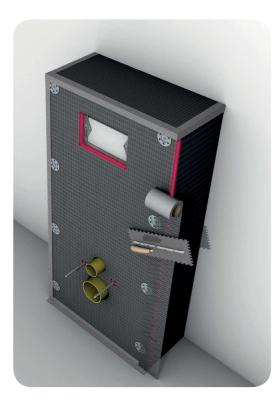
Apply q-glass-fibre tape and a thin coat of tile adhesive to all butt joints and edges.
