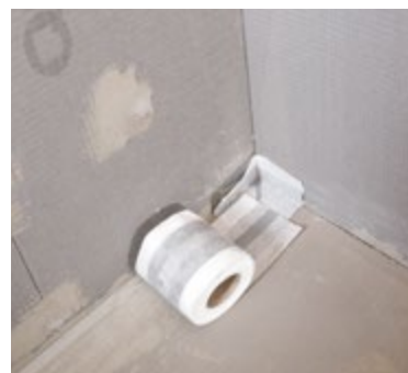
4. Seal all joints with Qboard® sealing set 2-k.
