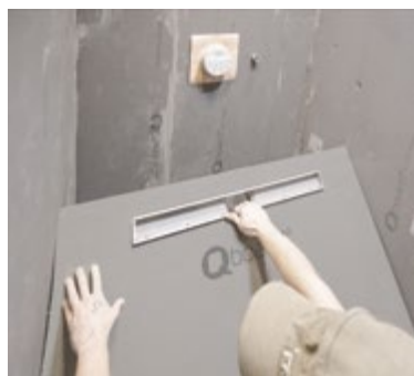
3. Apply adhesive to the entire surface of the shower element and bond to the hardened levelling screed. Use a tile or flexible adhesive for this.
