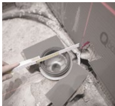
1. Connect the floor drain to the drainpipe and adjust the height.
