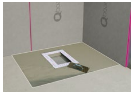
2) Fill the floor recess with leveling screed
