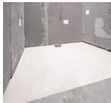
2. Fill in the screed recess with cement-based levelling screed and trowel it up to the corresponding height.
